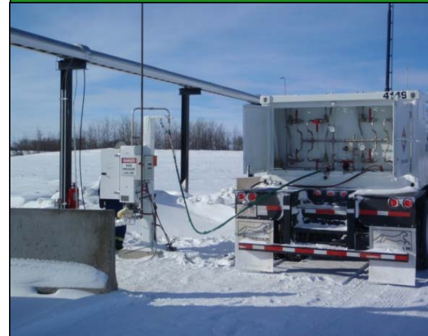
Unloading to Pipeline
